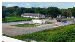
Fuel Storage Facility
