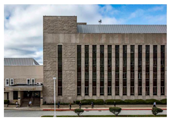
is in desperate need of a full building major renovation to abate asbestos-containing walls and flooring systems, replace deteriorating mechanical and plumbing systems, upgrade electrical and telecommunication systems, and install new life safety systems. The design for Phase 1 consisting of the basement and 1st floor was recently awarded in January 2022 with an anticipated construction award in FY24.
